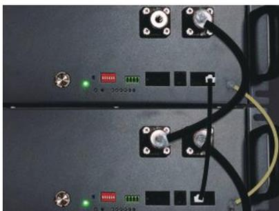
③ Connect the batteries with the battery communication wires.
